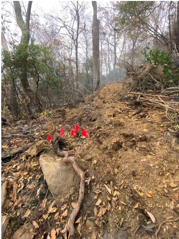
Photo #4 – View of “the rock” that cracked and caused the dozer to roll.
