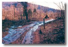
Temporary bridges, abutments, culvert pipes or other crossing structures should be removed prior to road closure. All stream channels should be restored to their natural condition.
